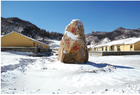
Unfinished houses of the Huangbaiyu demonstration village are visible behind a rock engraved with the characters "huangbaiyu" in red.
